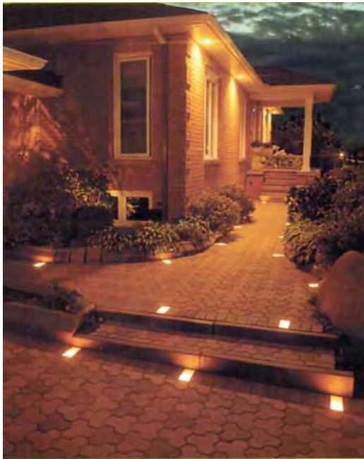
Sidewalk with 4"x8" pavers
