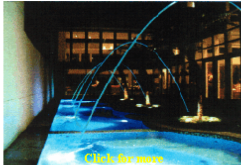
The laminar effect. A glasslike rod of water. See below for details.
